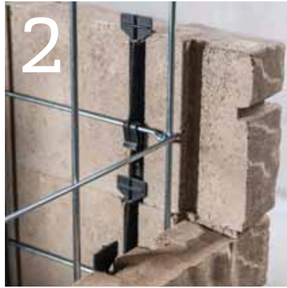
Use connector to attach Lafitt Tandem™ Ashlar Units to grid
